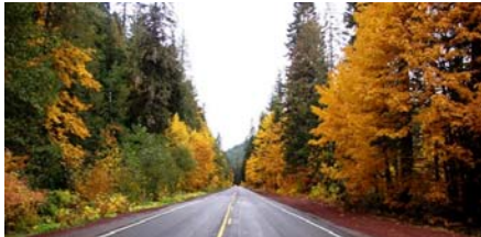
U.S. Highway 20 – West Side Photographer: Mike McArthur who stood on the center line to get the photo.
